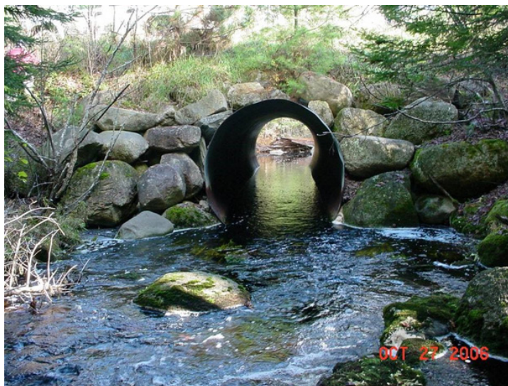
Road Crossing Before
